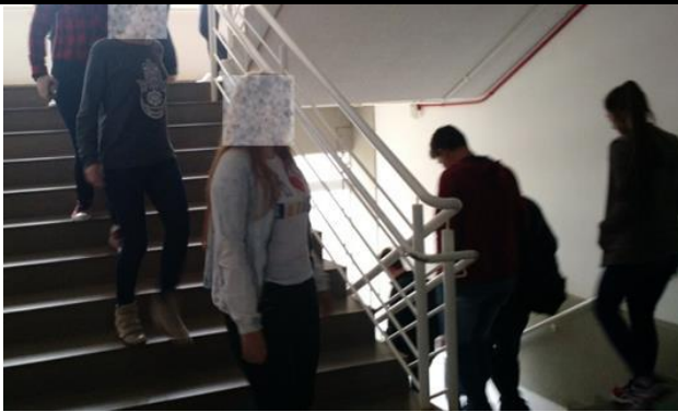
Fig. 4: Inside of the protected staircase 1
