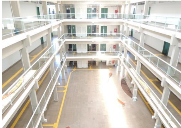
Fig. 2: Picture of the classrooms of Bloco A
