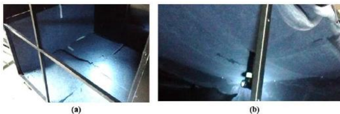
Fig. 10: Blankets application: floor and firewall (a) and ceiling (b)
